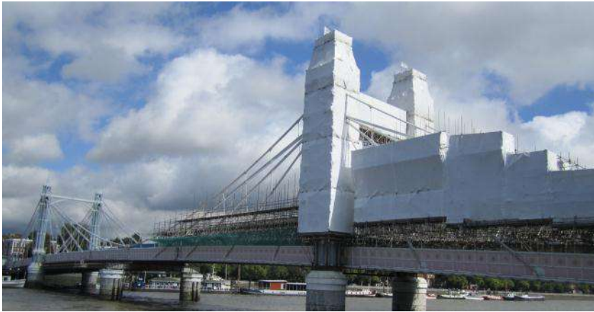
Albert Bridge under wraps during restoration
