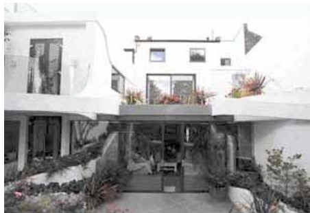
23 Mallinson Road, view from the back garden
