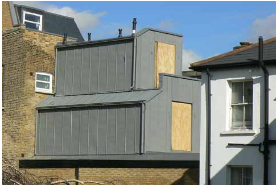
A view of a zinc extension from Frere Street
