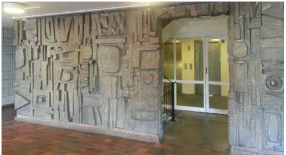
Striking sculptures on walls and entrances on the Winstanley estate, showcasing the materials used to build the estate in the 1960s
