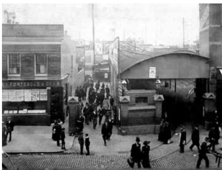
top Clapham Junction Entrance, St John's Hill c 1906, © Wandsworth Heritage Service above Marshall's Stables, Upper Richmond Road, 1897 ©Wandsworth Museum
