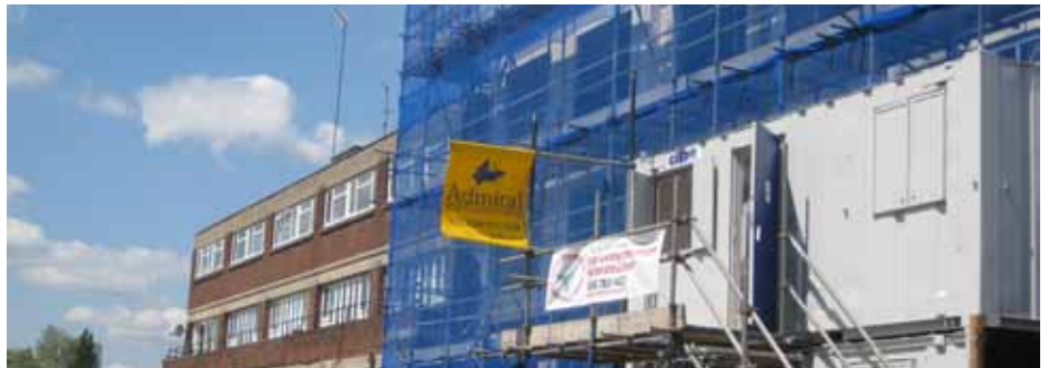
Roof lines need close monitoring in Chatham Road
