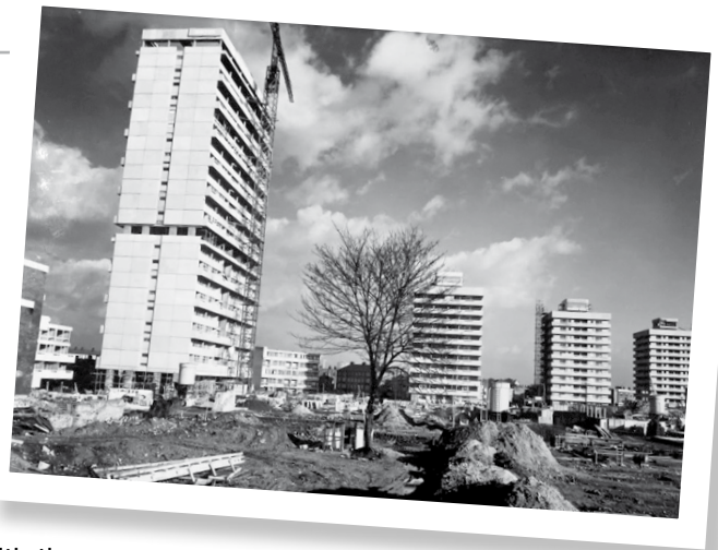
Above: Winstanley estate during construction. Below: a young interviewer at work
