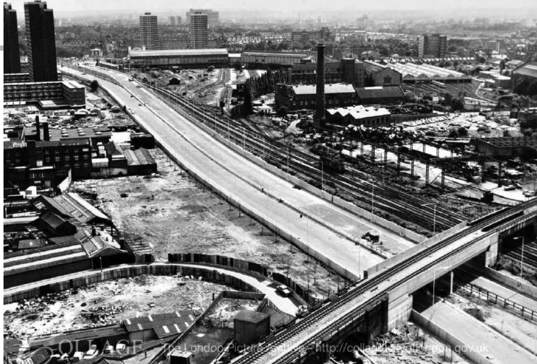
Ringway Westway under construction
